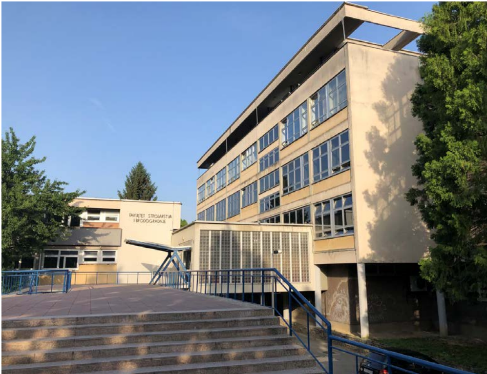
Nord building before reconstruction
