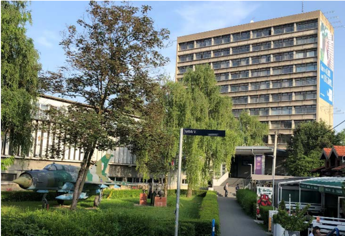
South building before reconstruction
